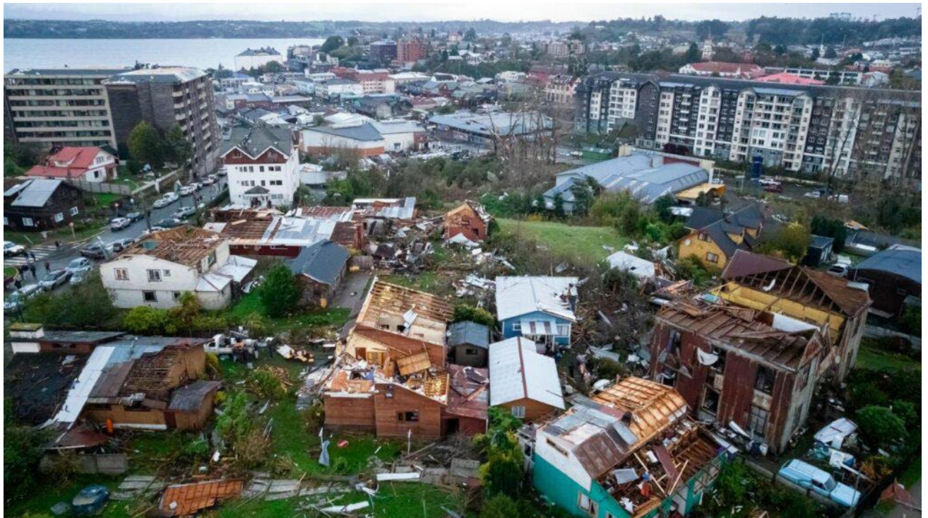
Figure 11 - Debris after the tornado struck the city of Puerto Varas on May 25, 2025, in the province of Llanquihue, Los Lagos Region, southern Chile (Source: UChile - Universidad de Chile)
